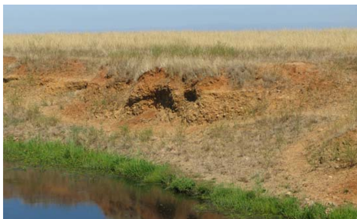
Erosion of the creek bank caused by livestock, Upper Laguna Creek.
