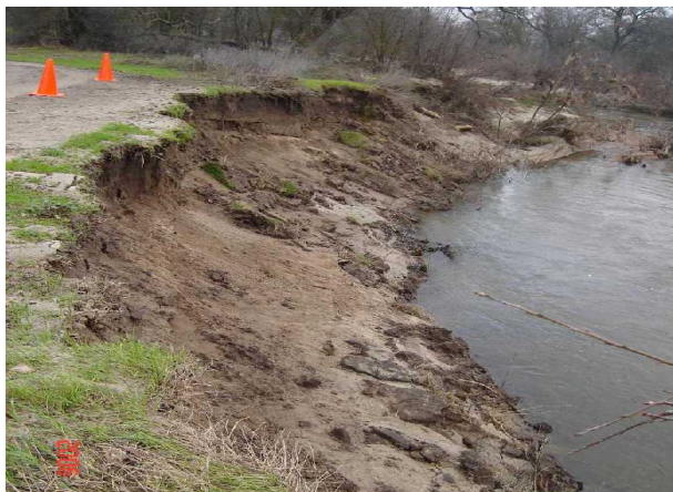
Classic signs of an ailing creek – eroded banks.
